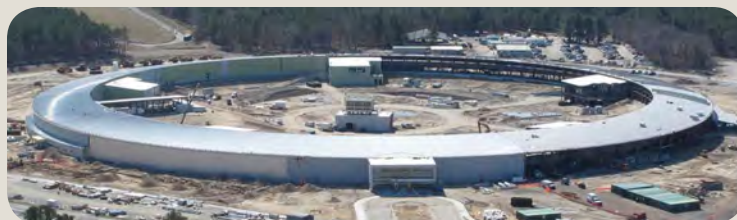
Fig. C1. NSLS-II under construction and ~50% complete on March 25, 2011. The new facility will produce photon beams with a brightness and coherence unsurpassed by any synchrotron worldwide and will support a wide range of experiments in the biological and physical sciences. [Courtesy of Brookhaven National Laboratory]
